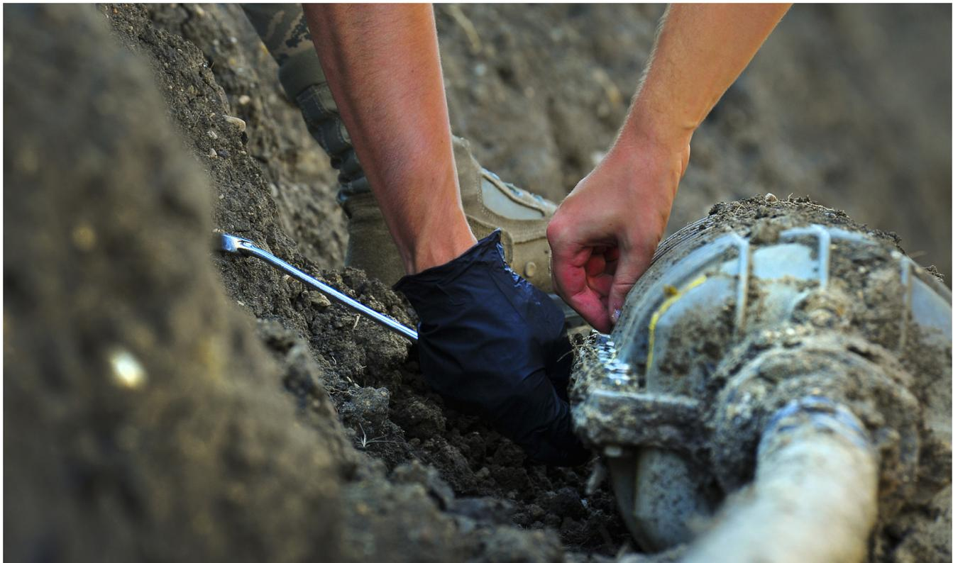
Airmen from the 91st Missile Maintenance Squadron Hardened Intersite Cable System section loosen the bolts on a splice case outside of a missile alert facility in North Dakota, July 31, 2014.
